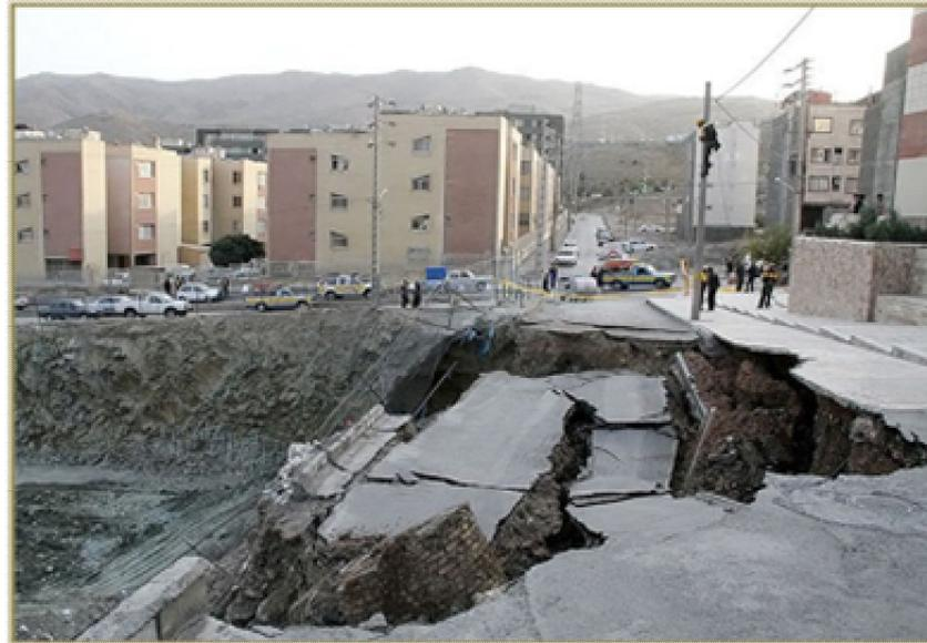
Figure 1. Excavation failure in metamorphic rocks of Hashemieh neighborhood in Mashhad (24/10/2013)
